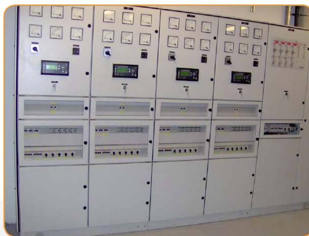
Styretavle for fire generatoranlæg, Glostrup Hospital. Foto: Scandinavian Engineering Systems A/S.
